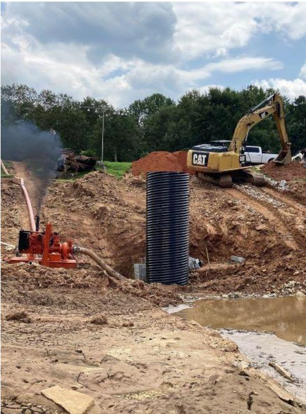
If you look closely at the picture to the left you might get a better understanding of what is happening. You can see black smoke from a pump that is removing lake water and sending it over the dam through a flexible pipe. You can also see a new load of dirt and at the base of the dam, cement blocks.
