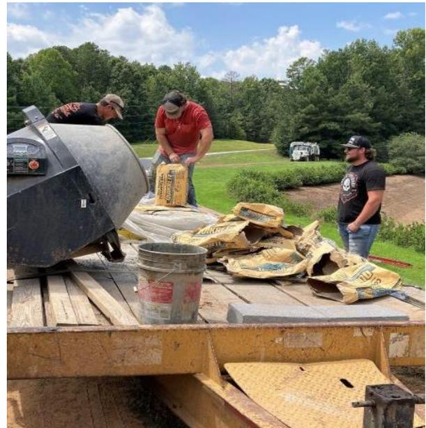
What Griffin Brothers has done is remove the old corrugated pipe and inserted the new high-quality pipe designed to last over 50 years. Earthen dams, like ours, are made from compacted dirt. So, there is now a need to replace the foundation of the dam with concrete blocks and cement. They are mixing cement in the picture shown above with the goal of reinforcing the foundation or floor of the dam.
