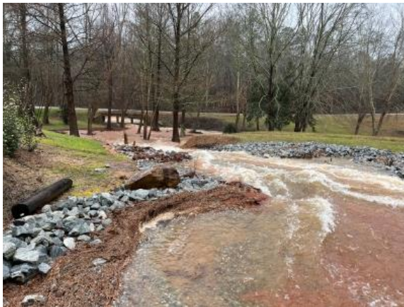
Water rushes into Creek crossing Hwy 335
