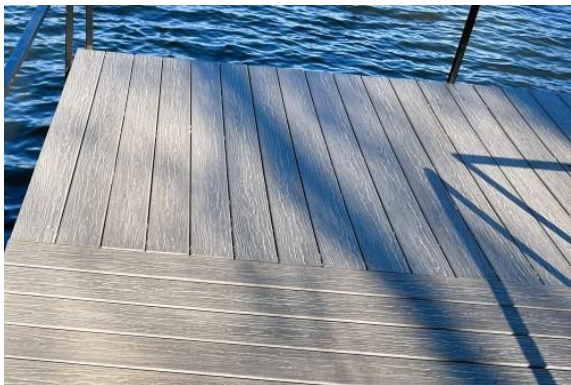
Moisture resistant materials on surface
