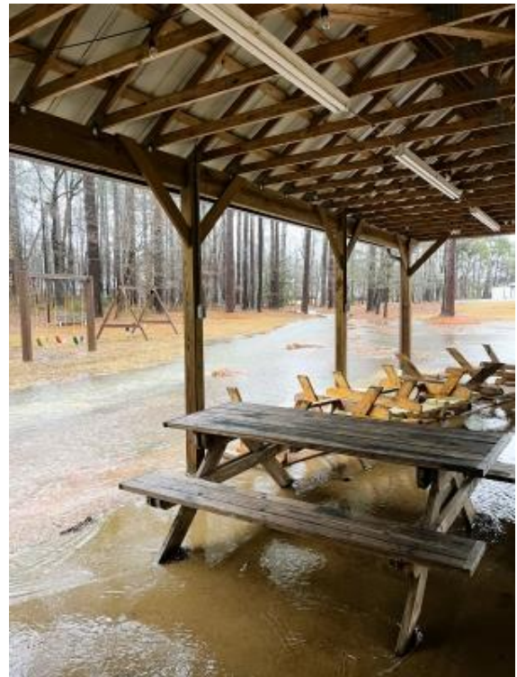
Water Rushes Past Recreation Center and Down Toward the Creek
