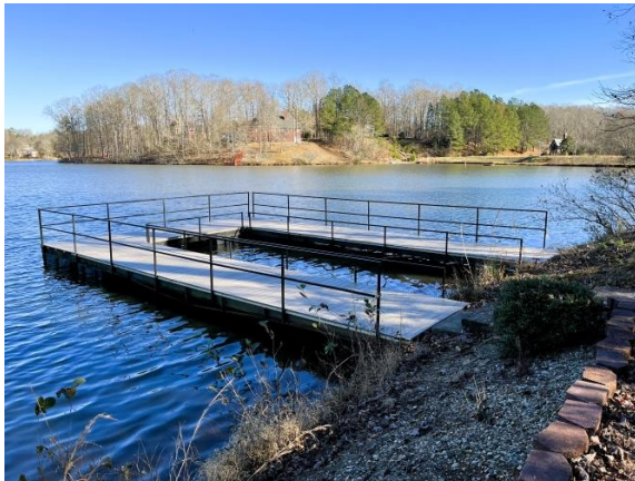
Upgraded Fishing Dock
